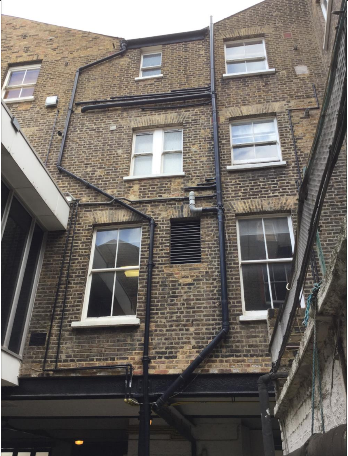
View of rear elevation from courtyard
