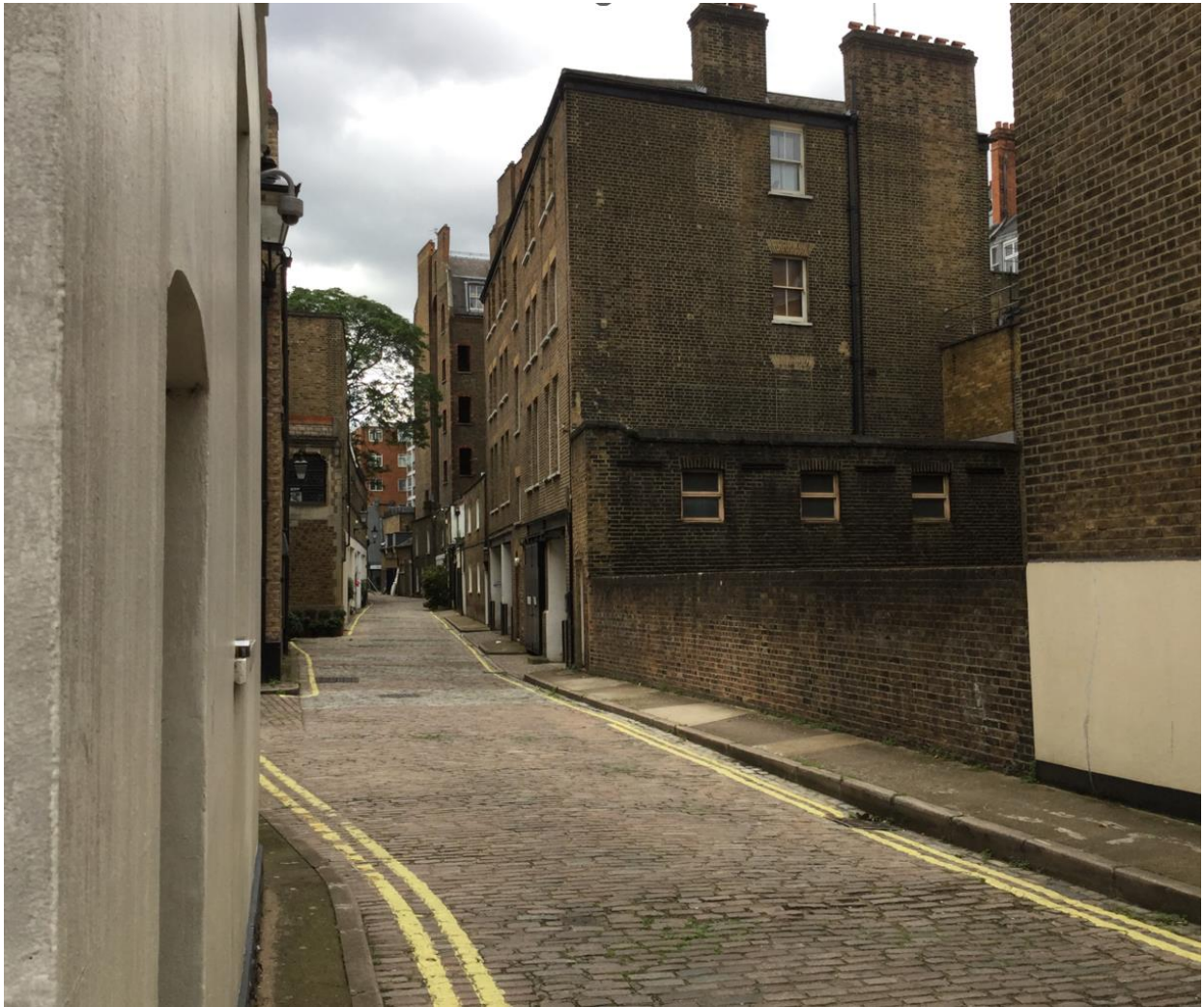
View and front and side elevation from Chapel Side near junction with Moscow Road
